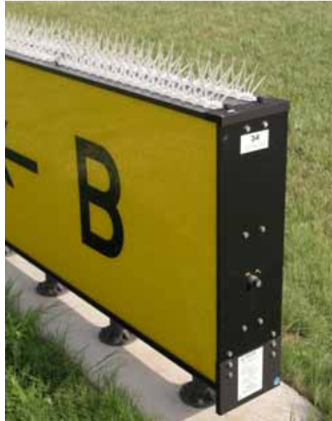
Figure 7. Bird anti-perching spikes fitted to the runway signage boards.
