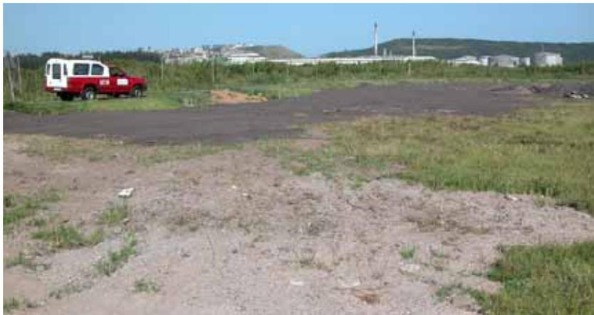
**Figure 6.** *An area where standing water collected has now been filled in with rubble and covered with soil.*
