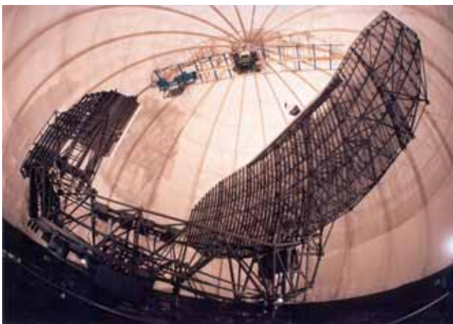
Figure 2. Inside view of the long-range air defence radar
